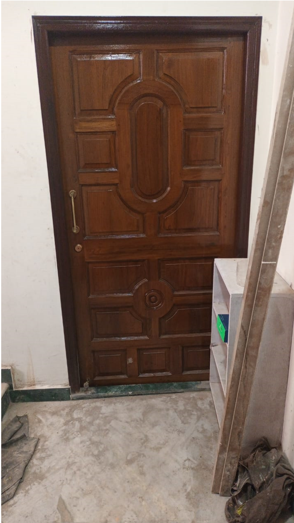
ASHA RESIDENCY_1 st FLOOR INTERNAL WORK COMPLETED
