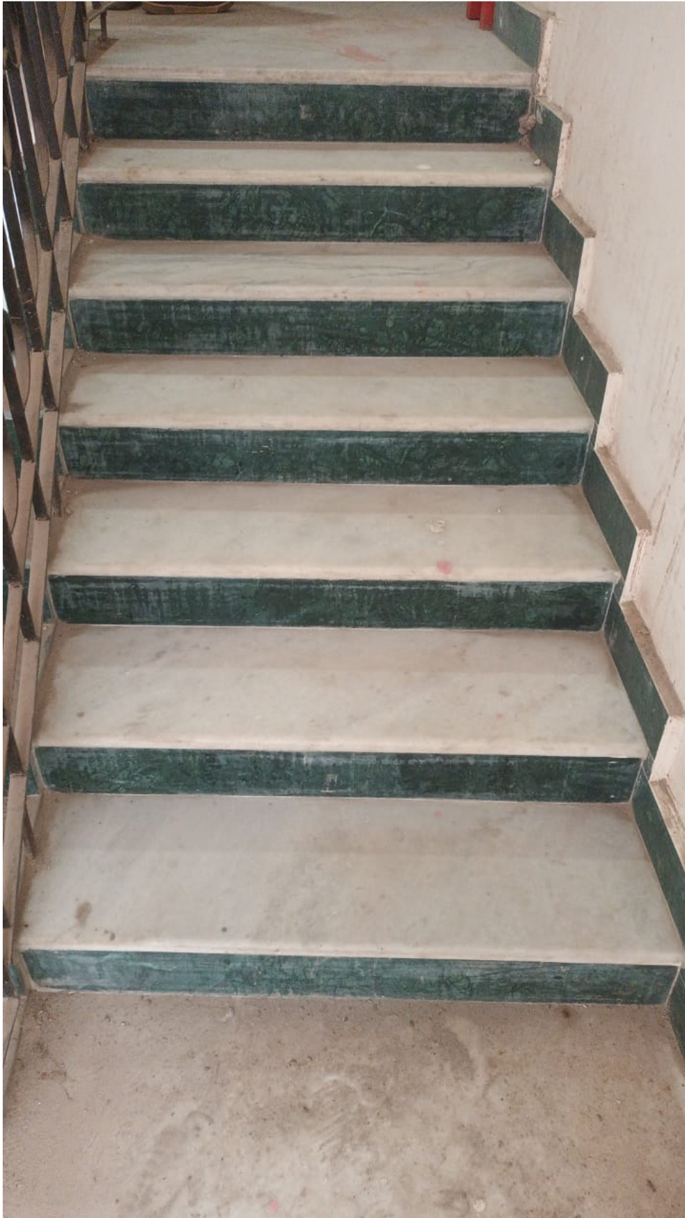
ASHA RESIDENCY_1 st FLOOR INTERNAL WORK COMPLETED
