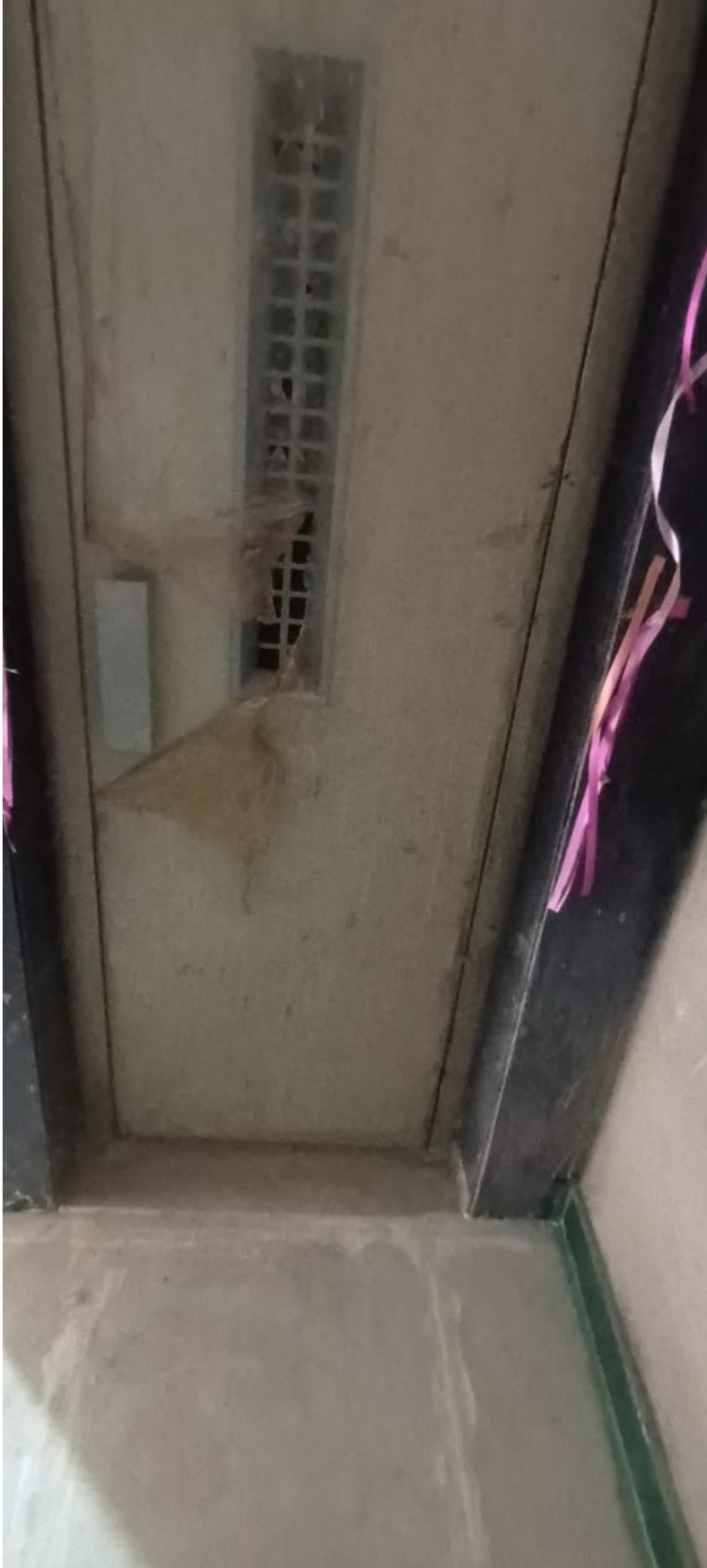
ASHA RESIDENCY_1 st FLOOR INTERNAL WORK COMPLETED
