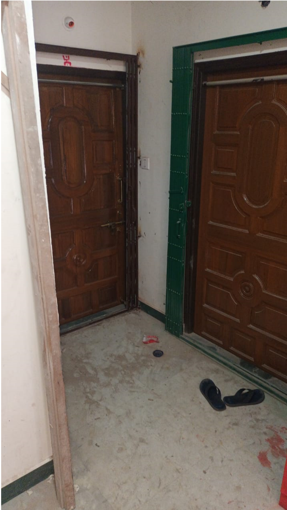
ASHA RESIDENCY_1 st FLOOR INTERNAL WORK COMPLETED
